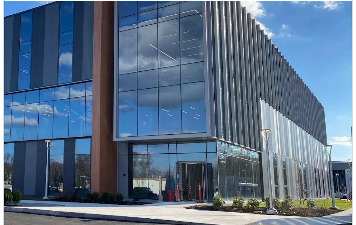
GT manufacturing facility in Bedford, MA
